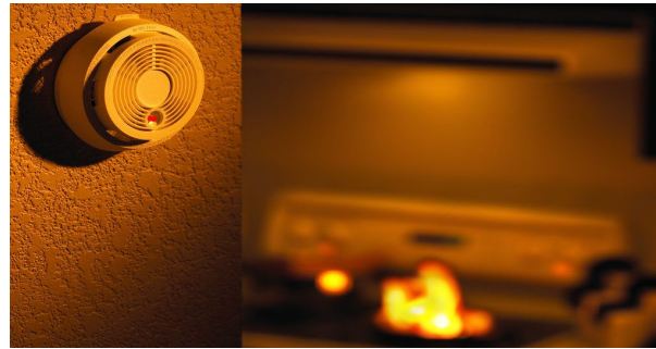
Fig. 6. Example of discrete smoke detector [7]
